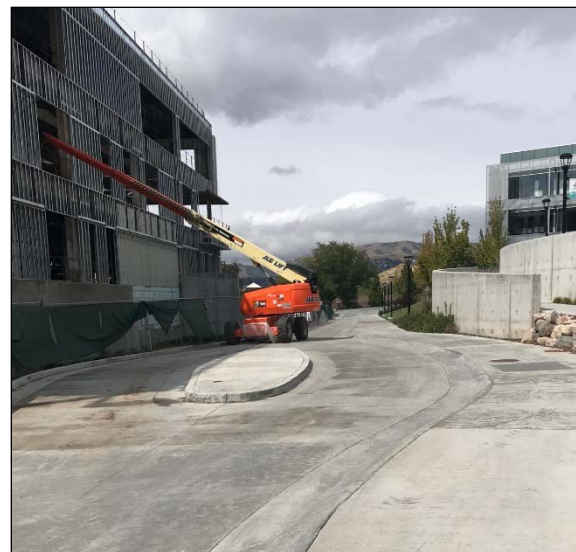
Figure 22. Rolled Curb at the University of Utah Busway
