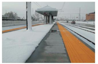
Testing Snow Melt System at Decker Lake
