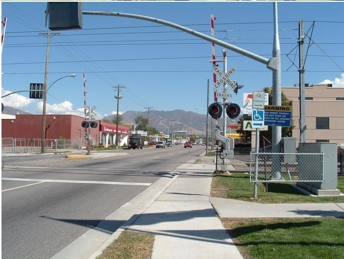
Figure 19-6: Example of Non-Exclusive Alignment with a Dedicated LRT Guideway
